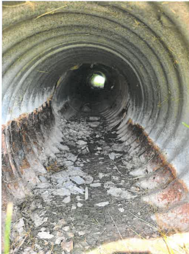
Driveway culvert looking west from east end of pipe.
