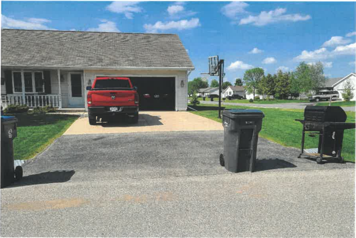
W5520 Colin St driveway apron.
