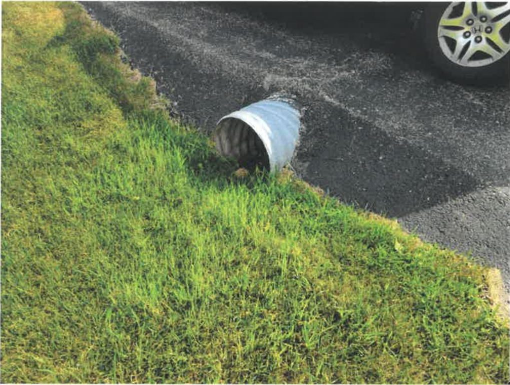
Western side of driveway apron.
