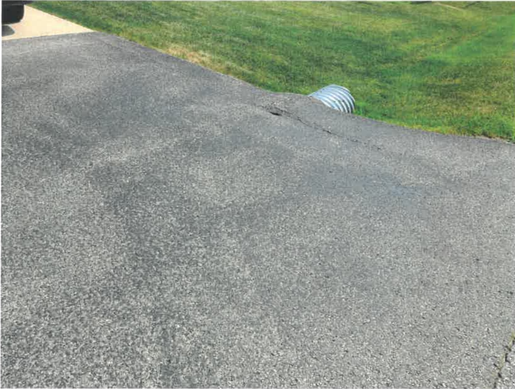
East side of driveway apron.
