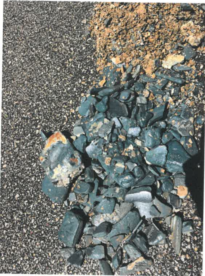
Mineral deposits removed from the mini-storm pipe.
