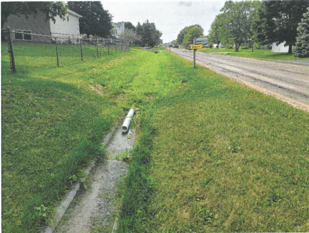
W6040 Coral Court Drain Tile Installation (Photos from 9-16-2020)
