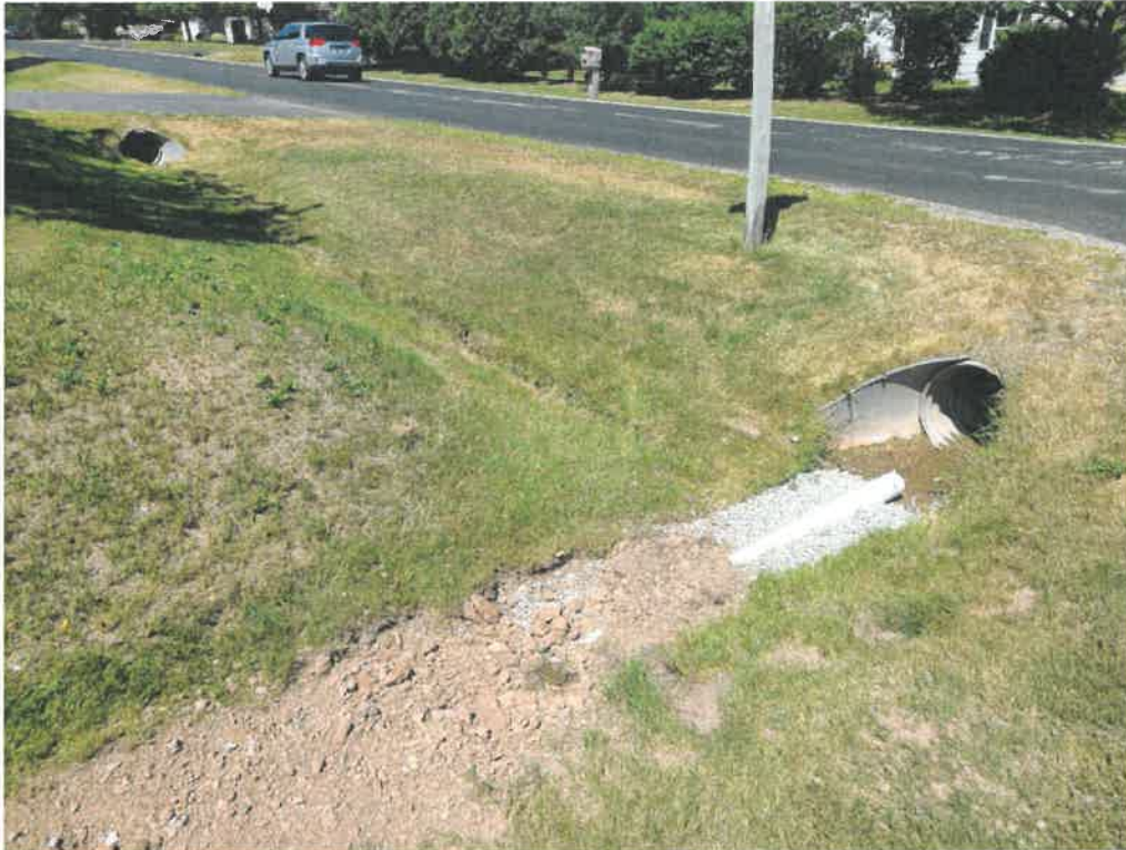
W5821 Hearthstone Drive Drain Tile Installation (Photos from 8-13-2020)
