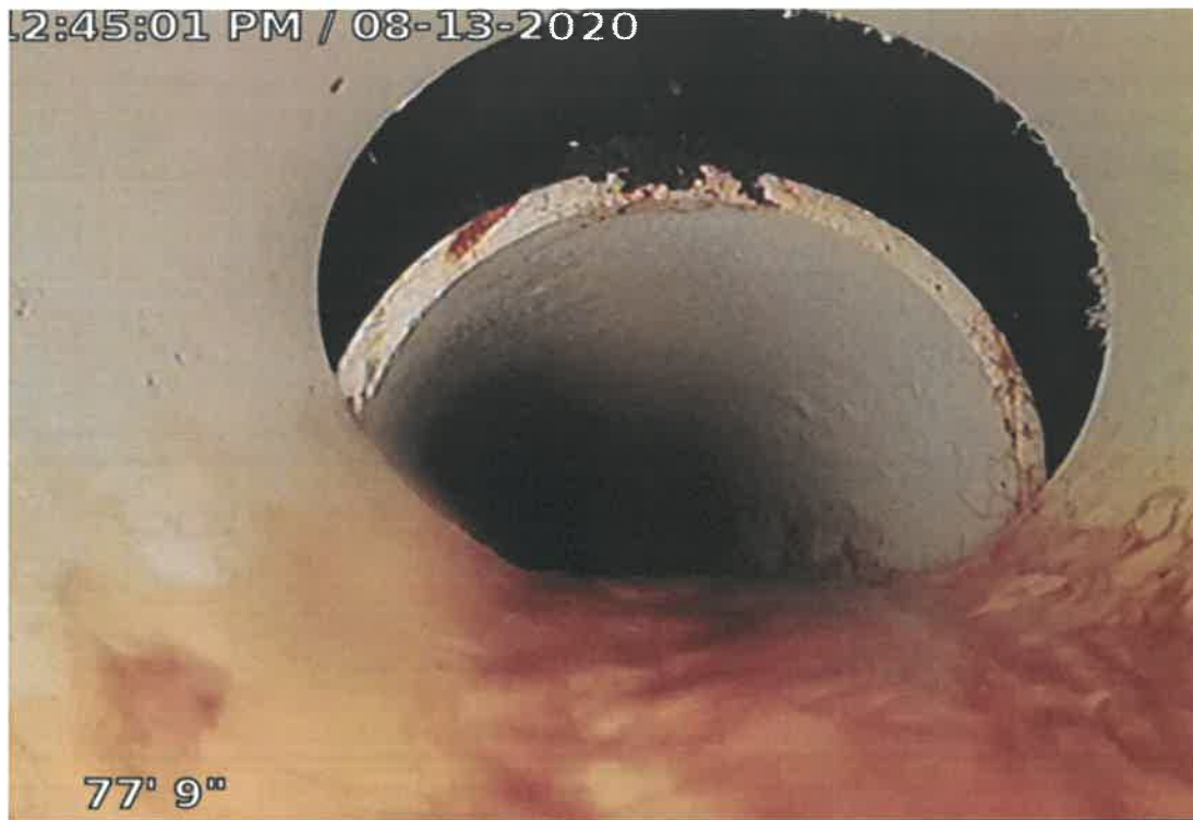
W5883 Augusta Place Pipe Offset
