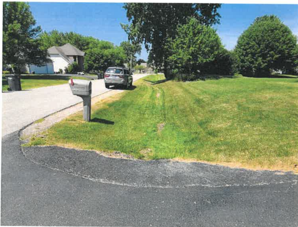
Looking west along the northern ditch of Augusta from W5878 Augusta driveway.
