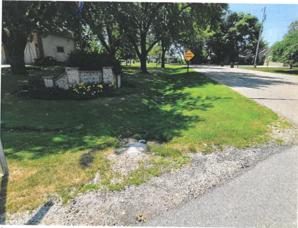
Looking south along the eastern ditch of Northshore at the Augusta intersection. This area had the most saturated ground on the entire section analyzed.
