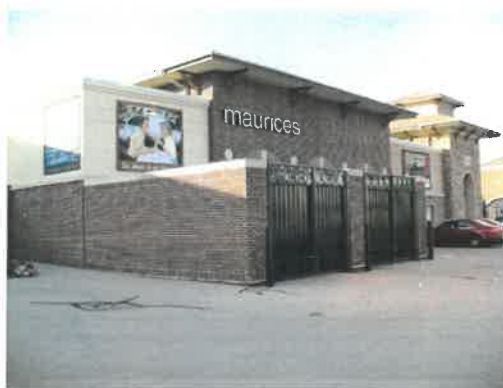
Outdoor storage facilities or waste receptacles require enclosure by a substantial screening system.
