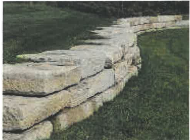
▲ Stacked limestone retaining wall
