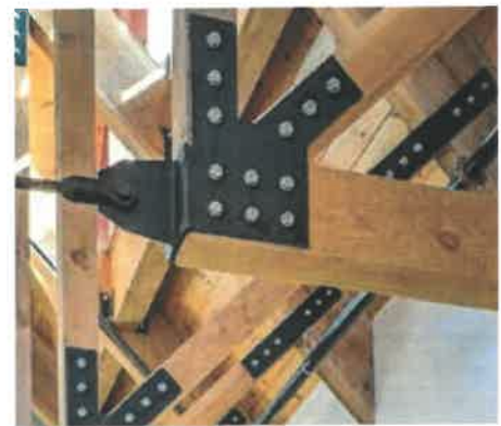
▲ Heavy timber with steel joinery. Source: vermonttimberworks.com
