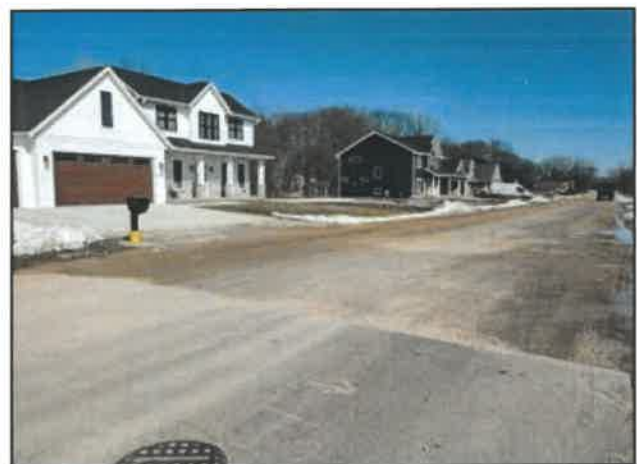
▲ An example of new subdivision construction in central Harrison, north of Lake Winnebago.
