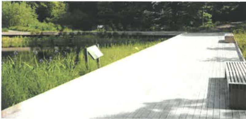
▲ Black Locust decking is a durable, sustainable wood for outdoor uses. Source: New York Botanical Garden
