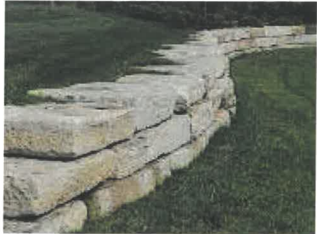
▲ Stacked limestone retaining wall
