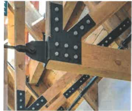
▲ Heavy timber with steel joinery. Source: vermonttimberworks.com
