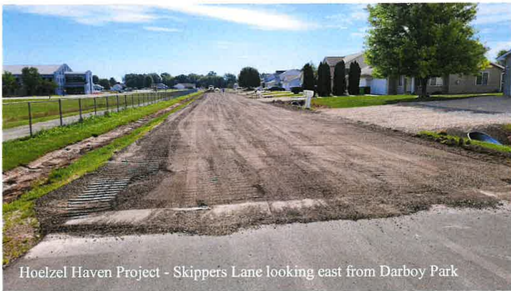
Hoelzel Haven Project - Hoelzel Way looking east
