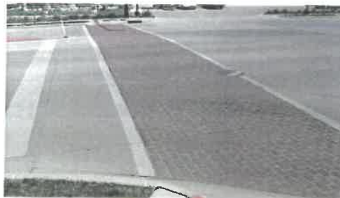
Special paving such as bricks, colored pavers, or colored brushed concrete to differentiate the crosswalks from the rest of the roadway.
