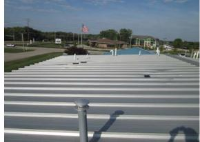
7. Deteriorating sealant at penetrations
