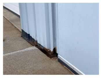
There was noticeable frost heaving of the approach slabs at the entrance doors. Over time, portions of the concrete was ground down to provide better accessibility to the entrances and eliminate trip hazards around the building.
