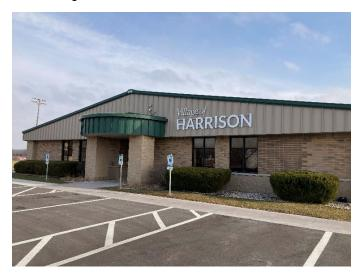
The parking lot contains concrete curbs and gutter around the South and West side of the building. Other areas of asphalt pavement are shouldered where they abut manicured lawn areas. Sheet drainage by sloping of the asphalt conveys stormwater away from the building. The asphalt parking lots have been recently re-paved and are in good condition.
