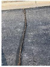
The parking lot contains concrete curbs and gutter around the South and West side of the building. Other areas of asphalt pavement are shouldered where they abut manicured lawn areas. Sheet drainage by sloping of the asphalt conveys stormwater away from the building. The asphalt parking lots have been seal coated and crack filled and are in fair condition.
