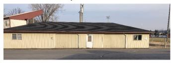
The North Face of the facility facing the ball diamonds remains open in the winter months. The construction of the concession building is similar to the toilet room facility. Vented aluminum soffits and prefinished metal fascia wrap the eaves. Wood roof trusses bear on exterior load bearing walls and the roof is comprised of wood sheathing and asphalt shingles. Drainage is conveyed by pitching the asphalt to a pre-formed asphalt channel that carries water around the building.
