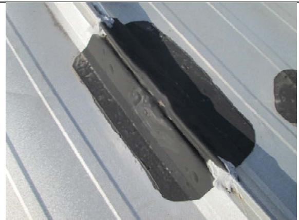
6. Panel repairs made with uncured EPDM and sealant
