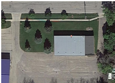
Site Aerial of Harrison Fire Station 60 W469 Clifton Rd, Sherwood
