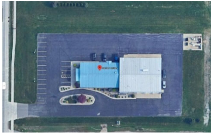
Site Aerial of Harrison Utilities N8722 Lake Park Road, Menasha
