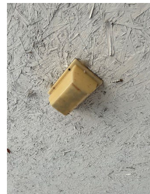
Existing Exterior Lighting Fixture
